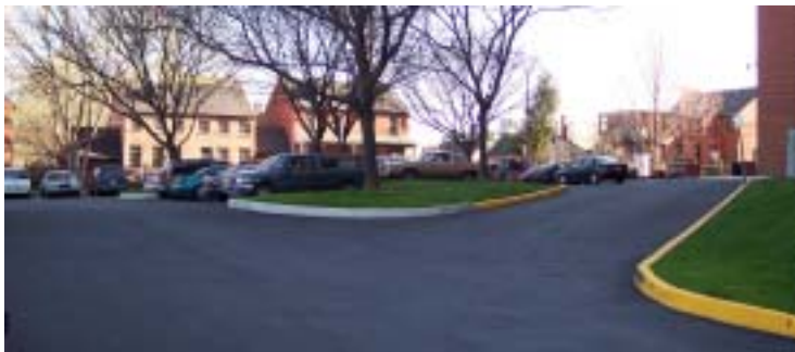
a repaved parking lot at Farnum Street East
