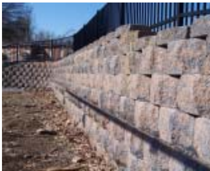
a new retaining wall at Franklin Terrace
